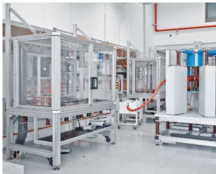
Fig. 25: Testing stations of the high-current testing system
