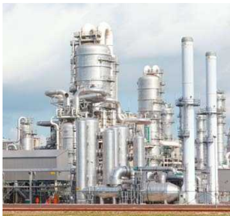
System expansion and post installation
