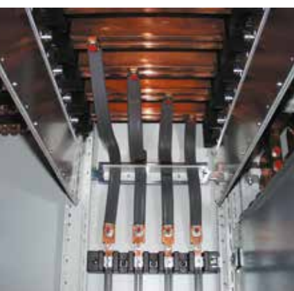
Connection: Busbar to busbar
